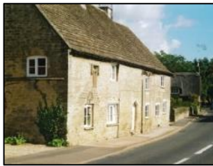
No. 7 Station Road
