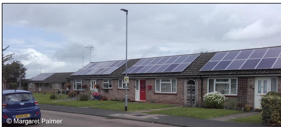
Solar panels on housing association bungalows, Little Northfields
